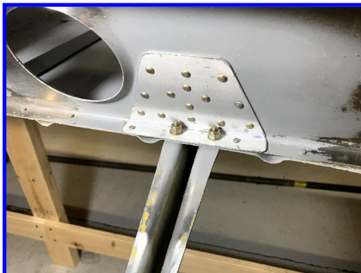
Completed patch with hinge hardware installed.
